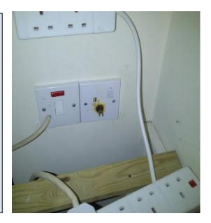
Extension leads should only be used as designed, and you should never 'daisy chain' extension leads together to overload the original plug and socket. If you use more than one extension lead per socket, it will significantly raise the risk of overloading the socket.
